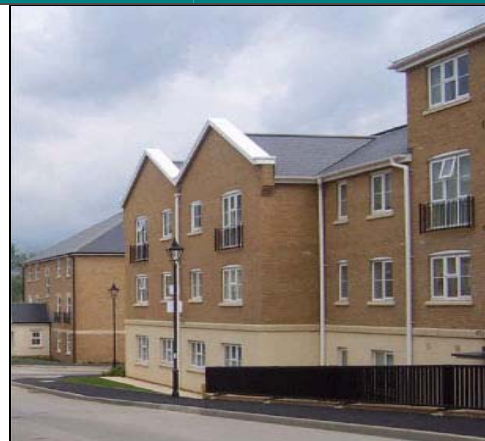
Affordable housing at Elizabeth Jennings Way
